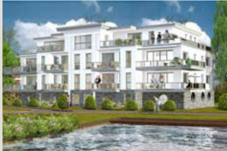
SEEBECKSTRASSE 15, BAD BEDERKESA
