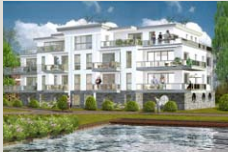
SEEBECKSTRASSE 15, BAD BEDERKESA
